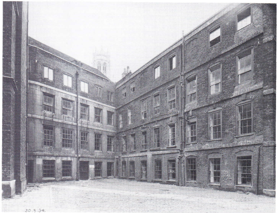
Looking south-west: the building no longer exists
